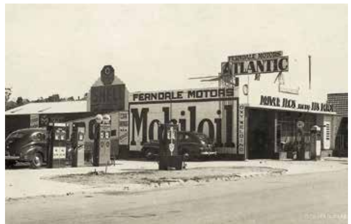
Driver Brothers Bus Depot and Service Station. 108/110 Glen Iris Road, Glen Iris circa 1948.
